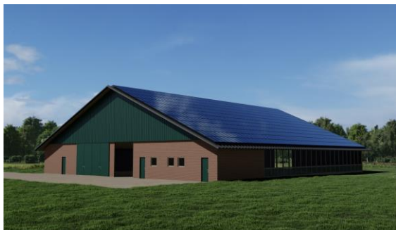
Figure 4. Dairy barn with rooftop solar panels
