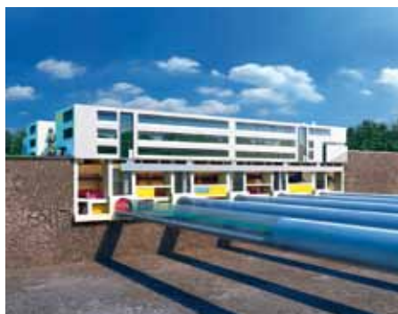
Montage of the main building with the underground experiment hall. (Copyright European XFEL GmbH)
